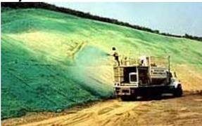
**Requirements:** Hydraulic mulches are recommended for temporary stabilization of areas with limited access. They can be after seed application or without seeding.
