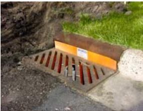
**Requirements:** All storm drain inlets must be protected by appropriate BMPs until all sources with potential for discharging to the inlet have been stabilized.
