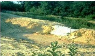
**Requirements:** Temporary sediment basins are recommended to retain sediment-laden runoff and allow sediment to settle out before leaving the site.
