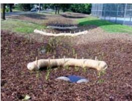
**Requirements:** Properly placed ditch checks are recommended for slowing water velocity in ditches.
