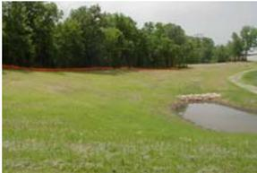
**Requirements:** If not being actively graded, positive slopes within 200' feet of a stormwater conveyance or water body must be stabilized within one to three weeks, depending on the slope. Temporary vegetation should be combined with mulch, erosion control blanket, or hydraulic soil stabilizers.
