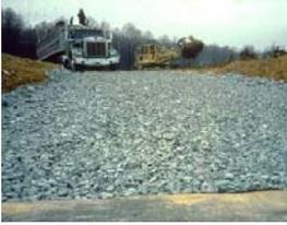
**Requirements:** Vehicle tracking of sediment from the construction site must be minimized by BMPs such as stone pads, wash racks, or equivalent systems.
