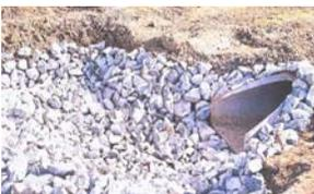
**Requirements:** Pipe outlets must have energy dissipation within 24 hours of connection to a surface water.
