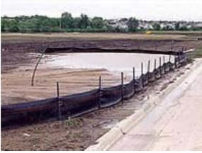
**Requirements:** Perimeter control is required before soil-disturbing activity begins. Silt fence is available as a standard woven geotextile or as a high-flow monofilament. It is designed to temporarily retain runoff and allow some sediment to settle out prior to leaving the site.
