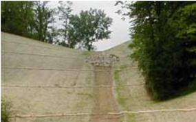
**Requirements:** Slope breaks are required every 75 feet on 3:1 slopes or greater.
