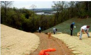
**Requirements:** Erosion control blanket is a recommended practice for stabilizing 3:1 and steeper slopes or the normal wetted perimeters of ditches.
