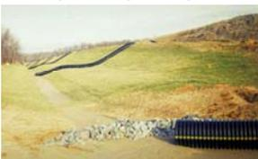
**Requirements:** Recommended for conveying runoff down sensitive slopes.
